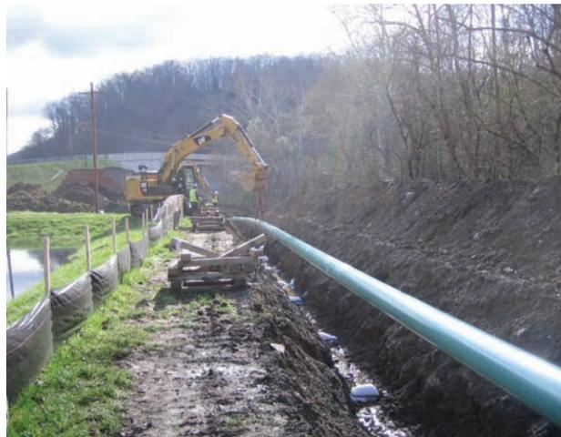
Pipe is lowered into the ditch on top of sandbags.
