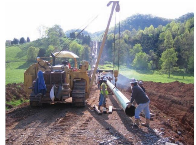
The ditch has been trenched and crews weld pipe in preparation for testing and lowering-in.
